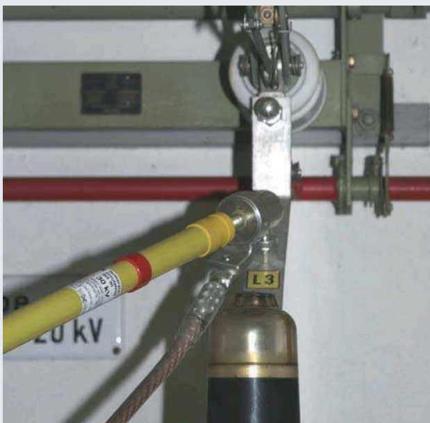
ISN SK insulating stick used for clamps with hexagon shaft of earthing and short-circuiting devices
