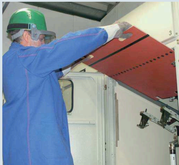
Inserting an insulating protective shutter (type A1) by hand
