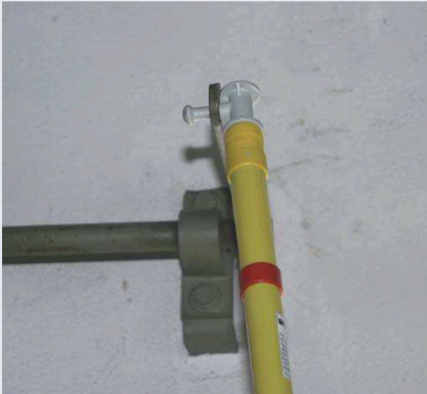
Switching a disconnector by means of an IS SK insulating stick fitted with switching stick head
